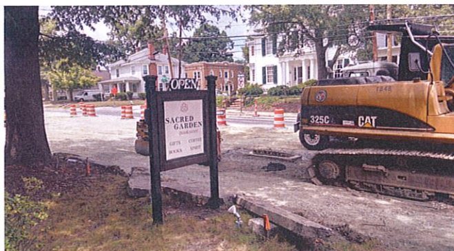
View from the Bookstore during construction
